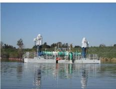
The original Santiago Pump Station was constructed at the bottom of Bond Basin in 2002. Four submersible pumps, each with their own MCC, were installed with varying power and head capacities to accommodate large fluctuations in water elevation. Soon after commissioning the station, three of the four pumps failed.
