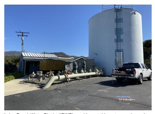
Irvine Ranch Water District (IRWD) provides potable water supply service to the Santiago Area located in an unincorporated region of Orange County. This service area includes four distinct sub-areas containing a system of reservoirs and pump stations that solely rely on the existing 150,000-gallon steel Zone 8 Fleming storage reservoir and the existing Zone 8 to 9 booster pump station as the main source of water supply.
